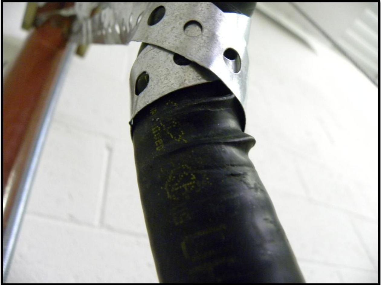
Figure 7. The deformation of the insulation resulting from the use of metal pipe straps
